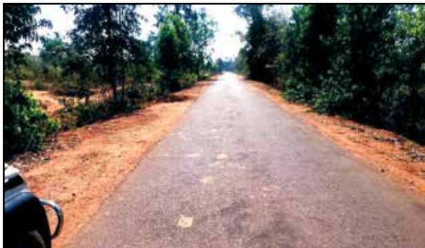
PMGSY Works at West Medinipur
