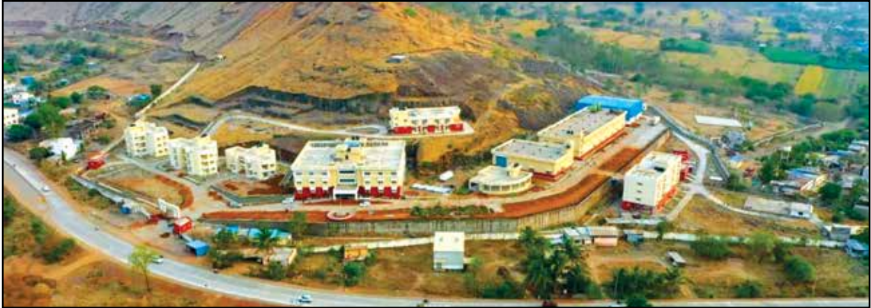
Construction of Seismological Research Centre for Ministry of Earth Sciences
