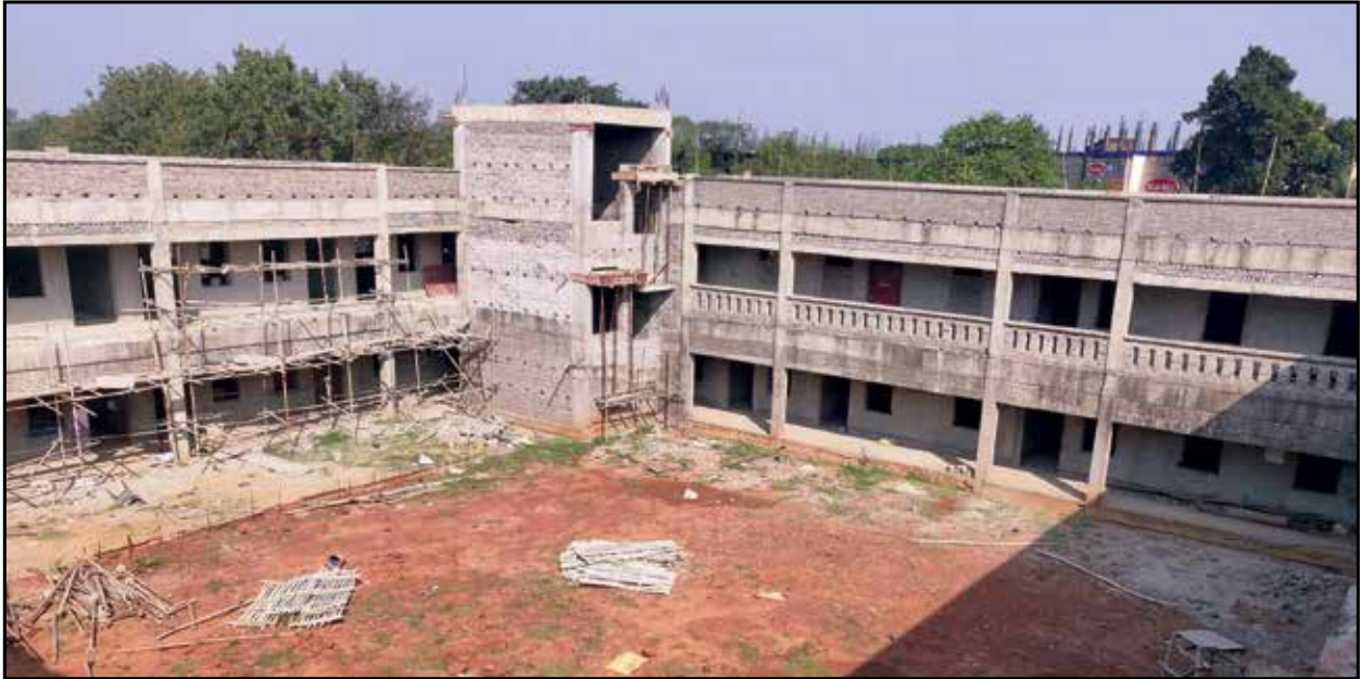
Construction of School Building at KVS, Kharagpur
