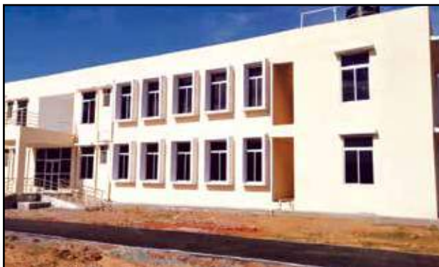
Construction of Eklavya Model Residential School, Bhalda, Mayurbhanj, Odisha
