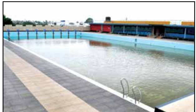
FINA Approved Stainless Steel Swimming Pool, Sports Authority of India, Aurangabad, Maharashtra
