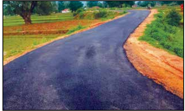
PMGSY Road Works of West Singhbhum
