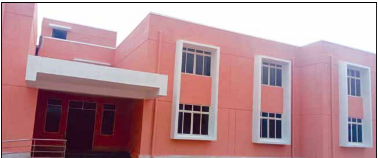
Construction of Post Matric 100 seated hostel, Baripada, Mayurbhanj, Odisha
