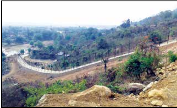
Eastern Border Fencing Work in Progress in Tripura
