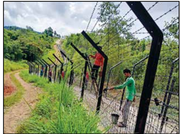
Fencing Work in Progress, Tripura
