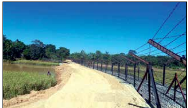
Indo-Bangladesh Border Fencing in Rajnagar, Tripura State
