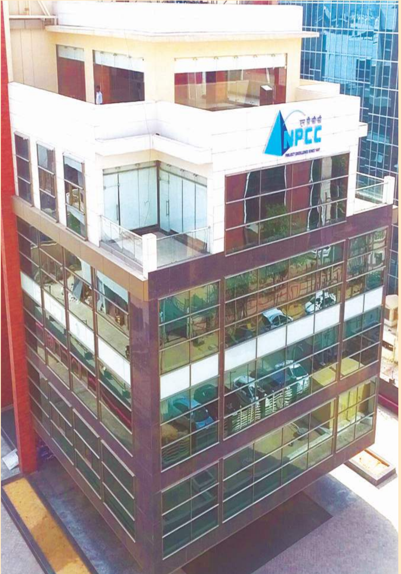
Corporate Office Building, Gurugram
