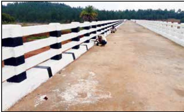
PMGSY Bridge works Gumla district
