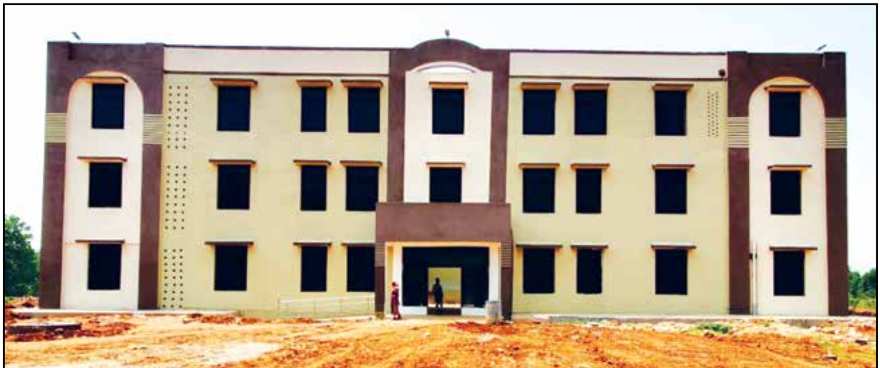
Construction of Eklavya Model Residential School, Telibani, Deogarh, Odisha
