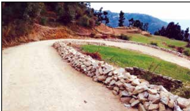
Road Works in Progress
