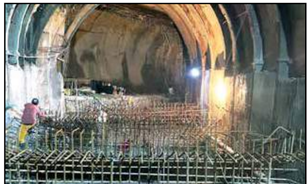
Adit Junction Head Race Tunnel
